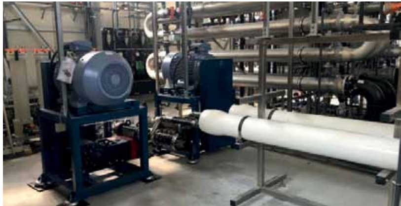
A Wannier Hydra-Cell pump in a reverse osmosis application.
